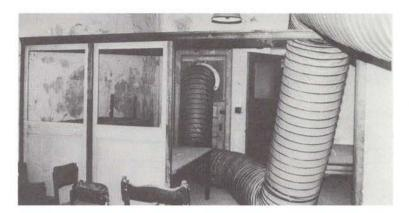
RESTORATION HEATING UP ON ELLIS ISLAND. Plastic ducts snake around and through the Main Building carrying heat to dry the moist brick and plaster walls. The project architects: BEYER BLINDER BELLE.
