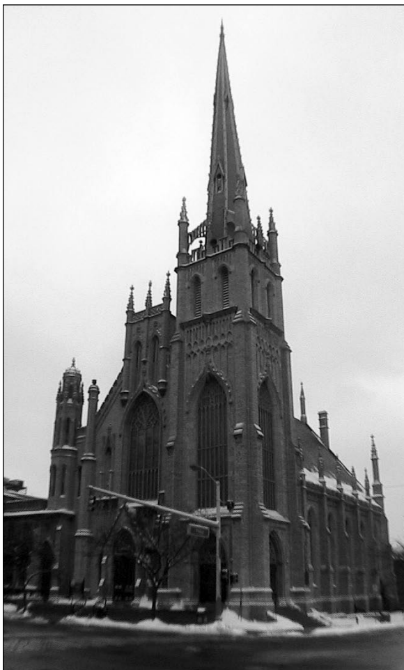
FORT STREET PRESBYTERIAN CHURCH, 1855, Octavius and Albert H. Jordon; 1876, 1914 (rebuilt)
