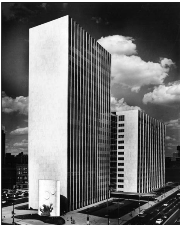
COLEMAN A. YOUNG MUNICIPAL CENTER (CITY-COUNTY BUILDING), 1955, Harley, Ellington and Day
